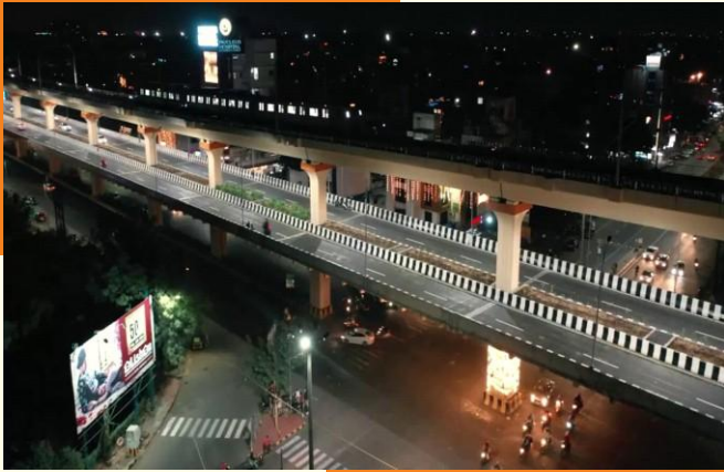
Double Decker Viaduct on Wardha Road-Nagpur
