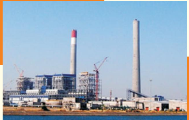
275 m high Chimney at KMPCL Subcritical Thermal Power Plant, Chhattisgarh
