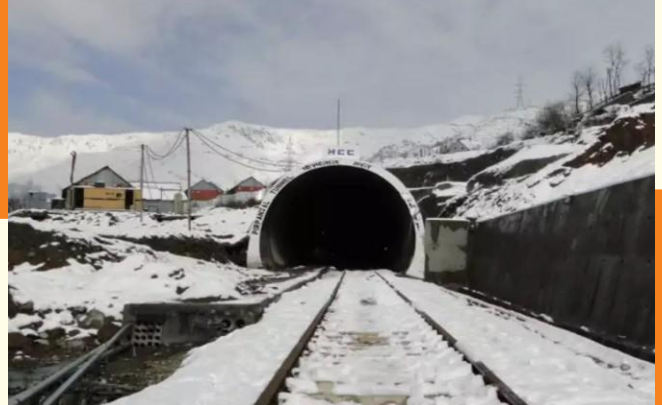
Pir Panjal Railway Tunnel - Jammu & Kashmir
