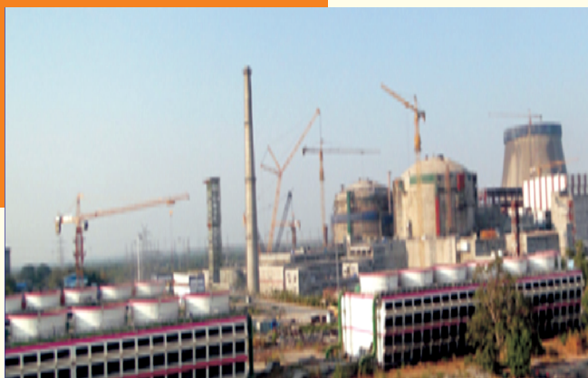
Kakrapar Atomic Power Project High Volume Fly Ash in Nuclear Reactor Dome Construction -Gujarat
